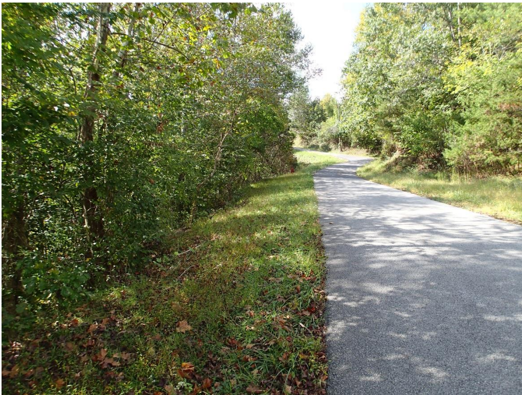
Figure 4-6. View of General Project Area: Circle Drive. Looking West.
