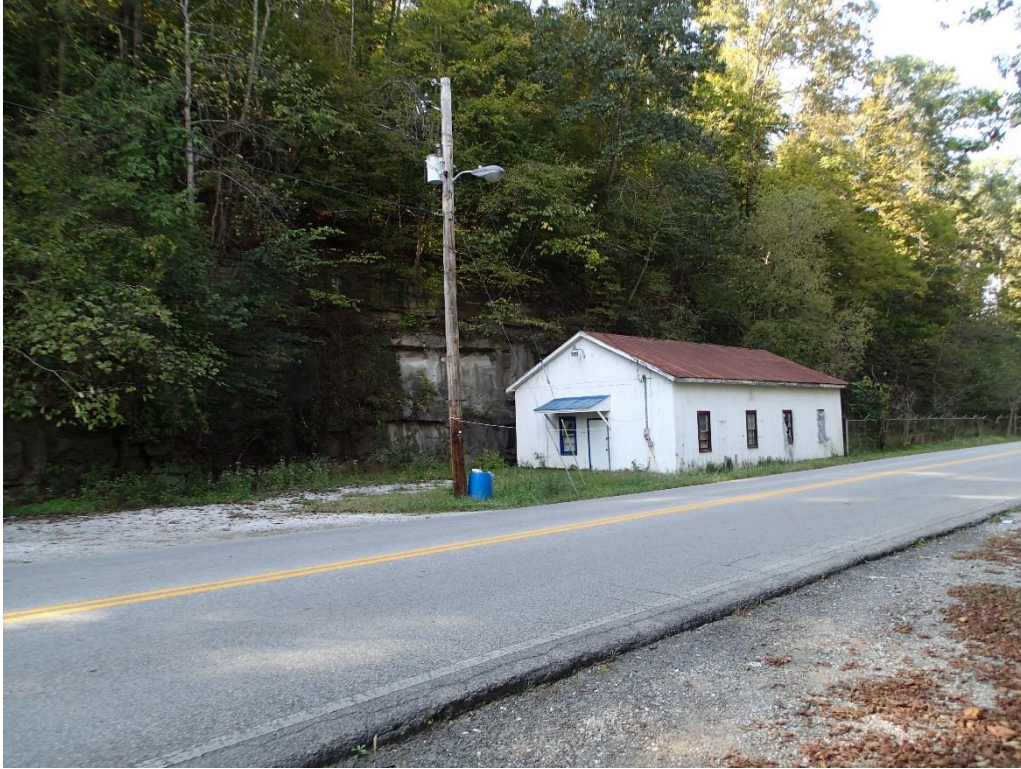
Figure 4-5. View of General Project Area: KY 2498 near US 460. Looking Northwest.
